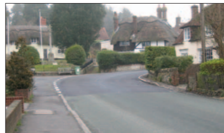
West Meon after some changes – removal of white lines, chevron and some signs. Change in road surface colour from green to black. (The black will be buff coloured when the project is finished).
